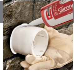
Caulk wall opening.
